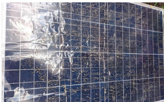
Fig.5 - Solar panel with dirty film
